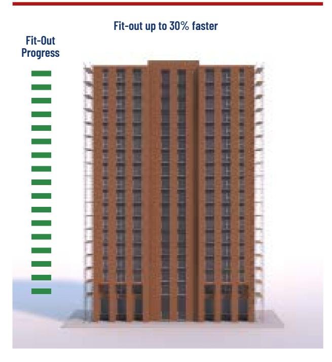
THIS CIRCUMVENTS THE CONVENTIONAL REQUIREMENT TO TOP OUT THE BUILDING AND CREATE A COMPLETE DRY ENVELOPE BEFORE COMMENCEMENT OF FITOUT BEGINS AS WITH TRADITIONAL REINFORCED CONCRETE BUILDS. THE BRICKWORK IS ALSO REMOVED FROM THE CRITICAL PATH FOR FURTHER PROGRAMME BENEFITS.
